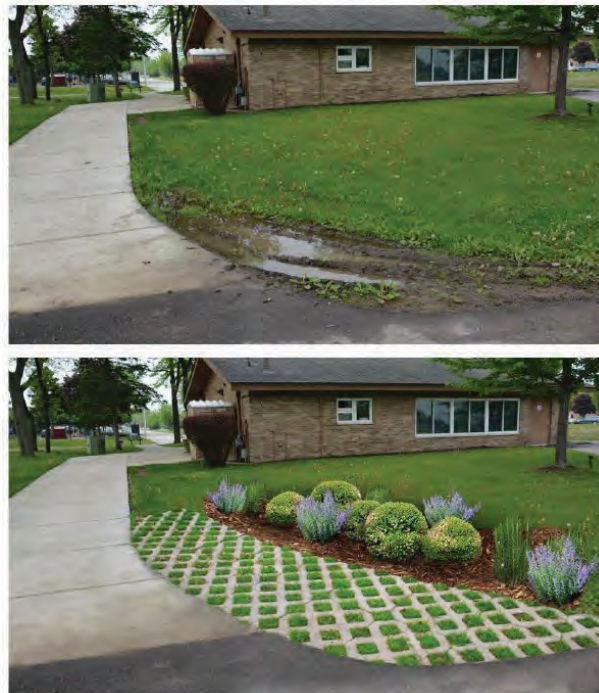
Figure 2 – Reinforced Pavement Edge Example
