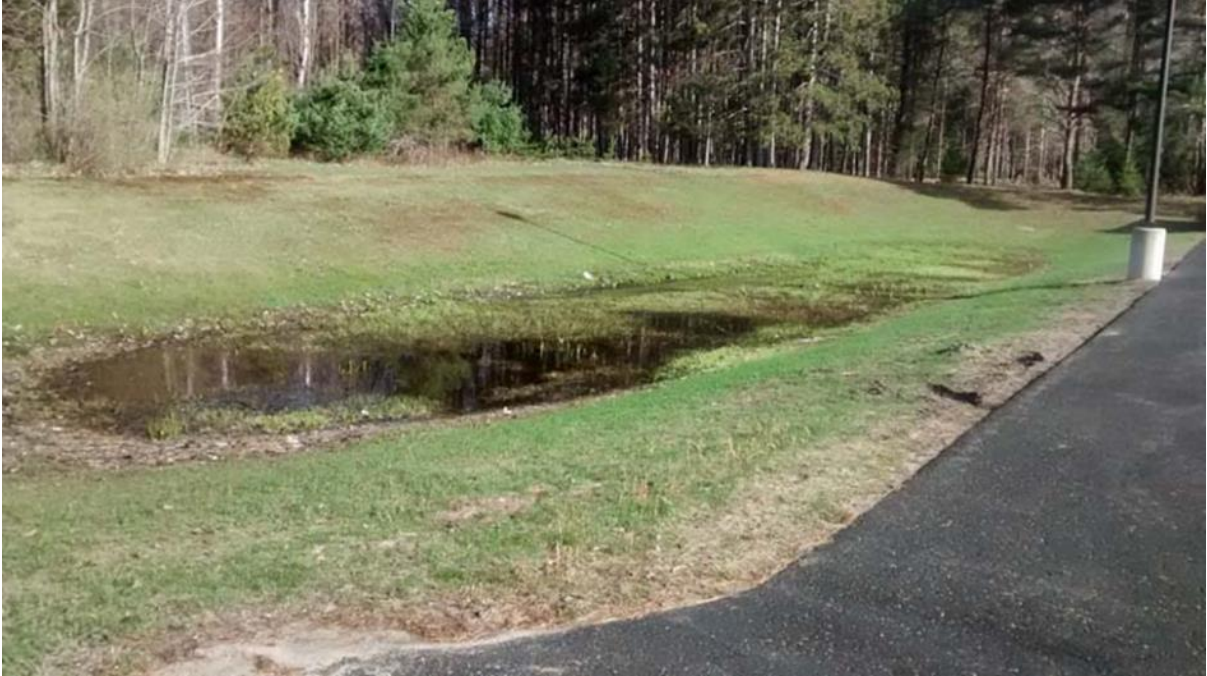
Figure 72: An infiltration basin at the Alanson Fire Station development (TOMWC)
