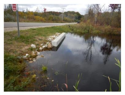
Figure 12. The new concrete box culvert on Fineout Creek/E. Shadow Trail
