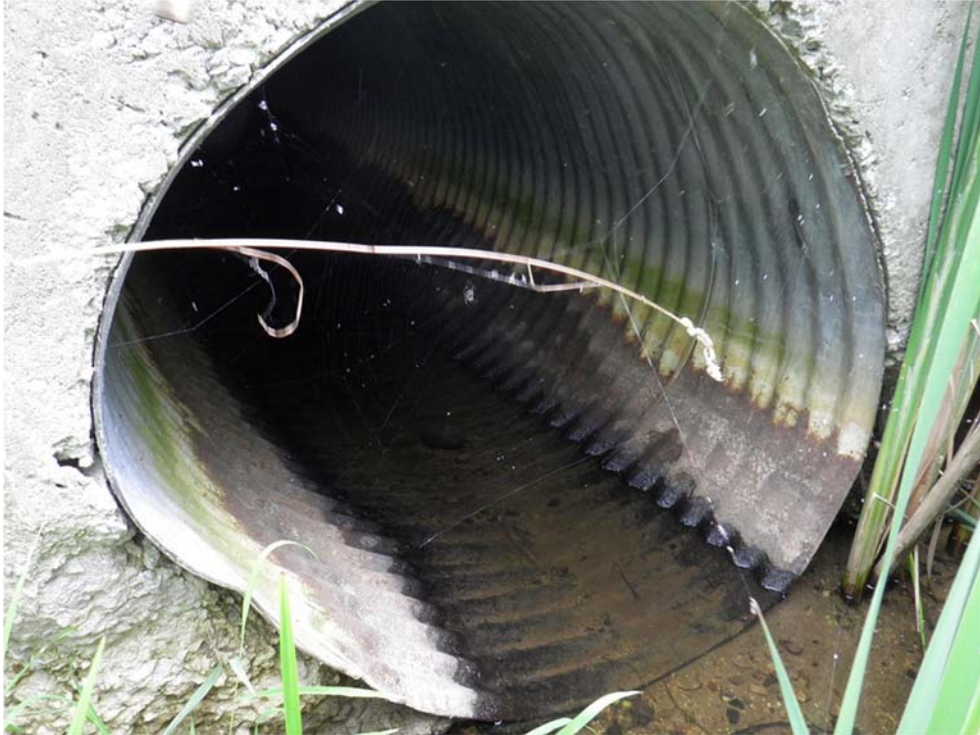
Figure 20: Butler Ditch culvert under Butler Rd. (DG 01)
