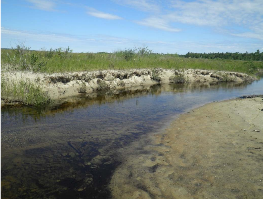
Figure 23: Erosion on Elliot Creek (DGB 02)
