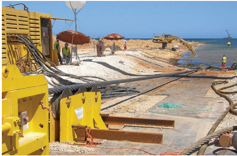
Figure 18: Pull wire set up for typical open cut shore crossing.
