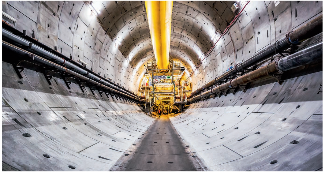
Figure 5: Precast concrete lining in the completed Eurasia Tunnel project in Istanbul. (Source: Herrenknecht)
