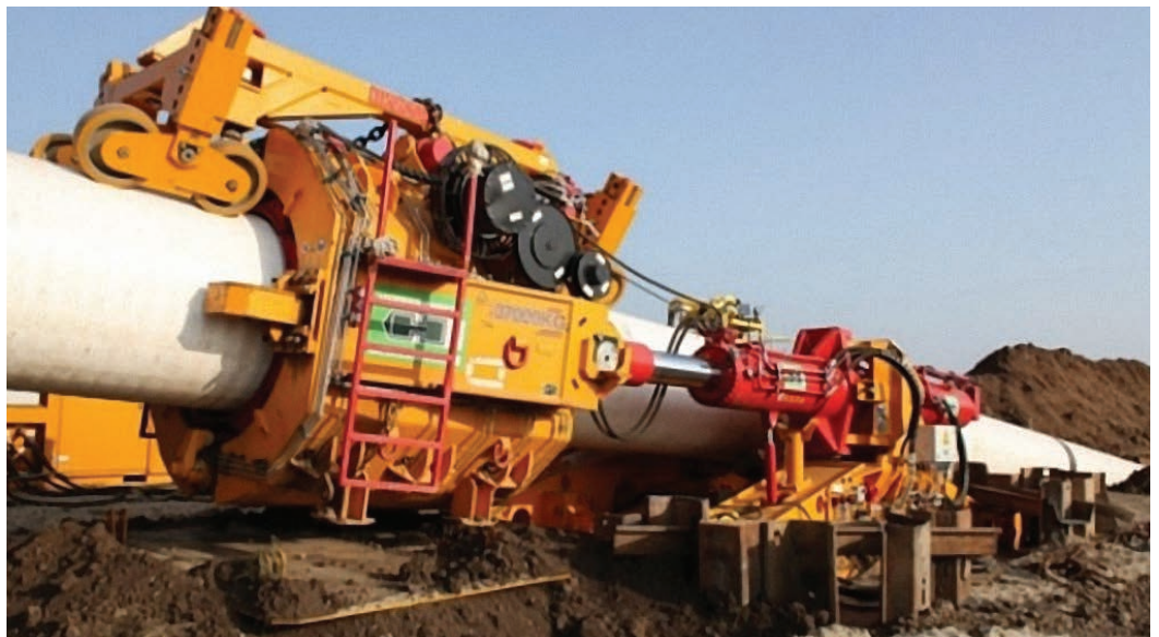
Figure 6: A pipe thruster pushing pipe.
