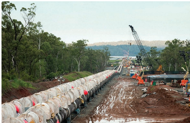
Figure 19: An onshore pipe staking set up.
