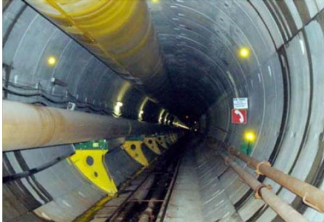
Gastau tunnel (17.5 ft internal diameter)
