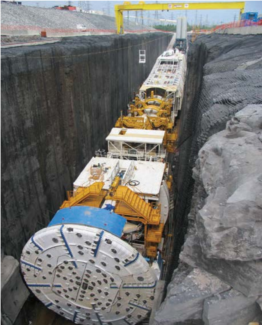
Niagara tunnel portal (45 ft diam. TBM)
