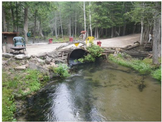
Culvert inlet and scouring pool on private road on Cold Creek.
