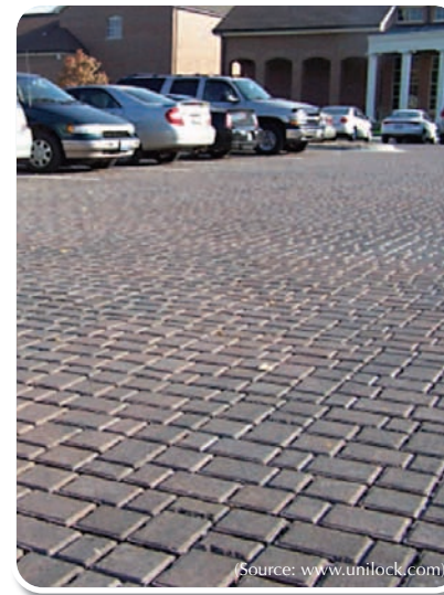
Parking lot with permeable interlocking pavers. (Source: www.unilock.com)
