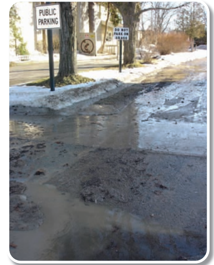
Sediment laden stormwater runoff from Charlevoix public parking lot.
